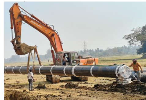
Lowering of Slurry Pipeline in Odisha
